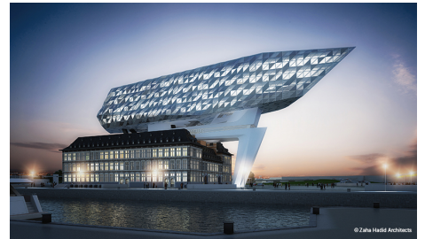
Technical installations in buildings
